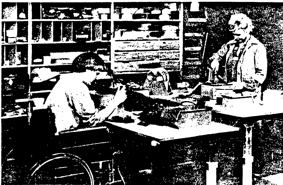
Fig. 44. An adjustable device for lowering the working plane for use in a standing or sitting posture. (Photo by courtesy of the Swedish Institute for the Handicapped)
