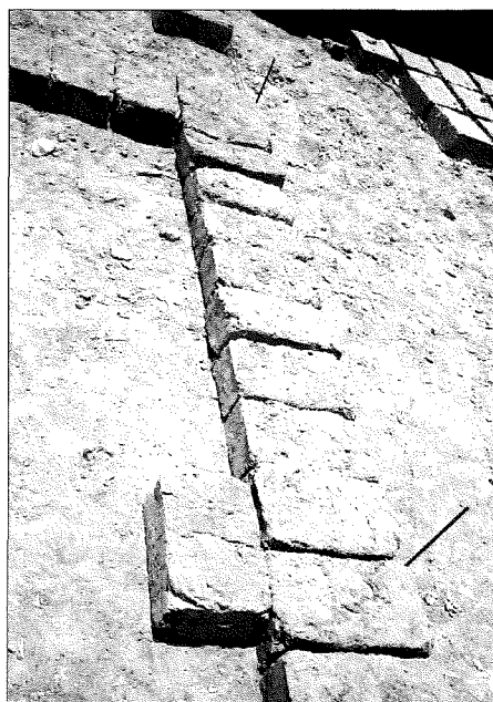
Figure 1 Ordinary mud bricks of local dimensions are used as the unit of measurement in laying
