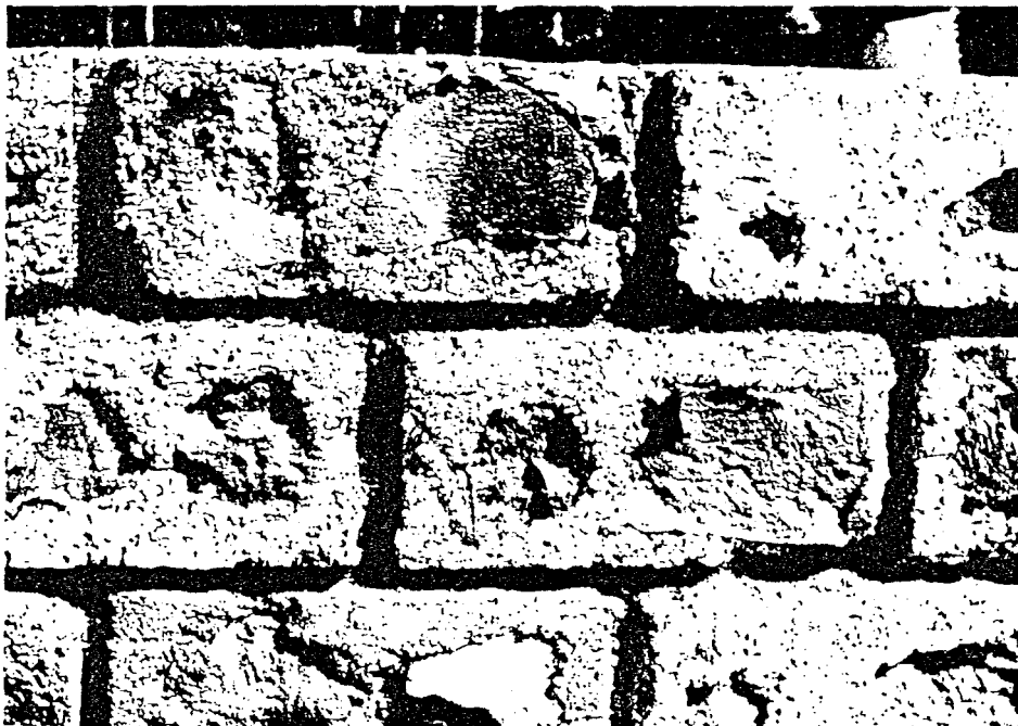
Stone block masonry walling.
