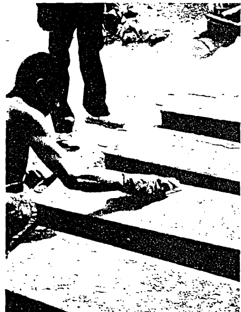
Fig. 7. Finishing tops of blocks.
