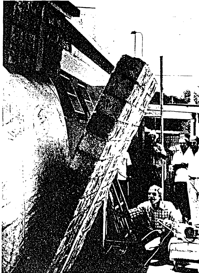
Unreinforced stone masonry wall at the time of collapse.
