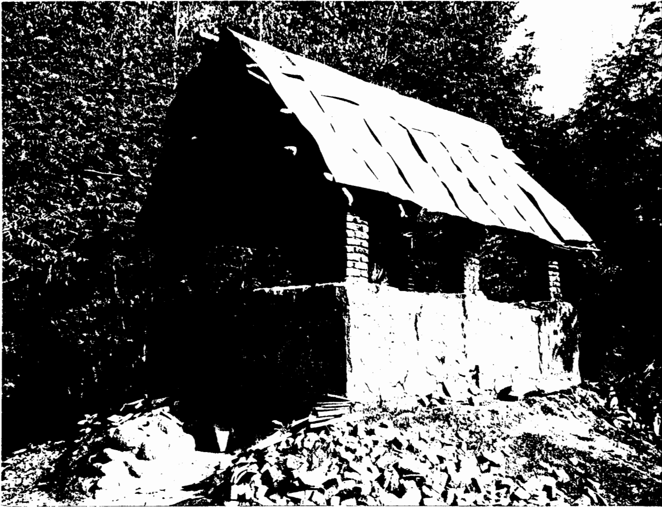
Chubar open top updraught kiln with capacity of 7500 tiles.
