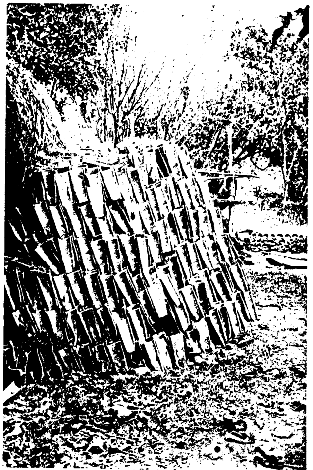
Method of storing fired tiles.
