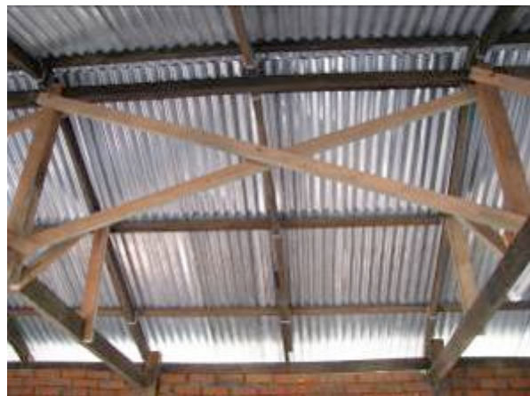
Diagonal Bracing bet: trusses
