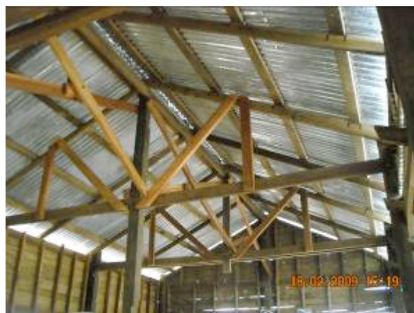
Bracing in & between trusses
