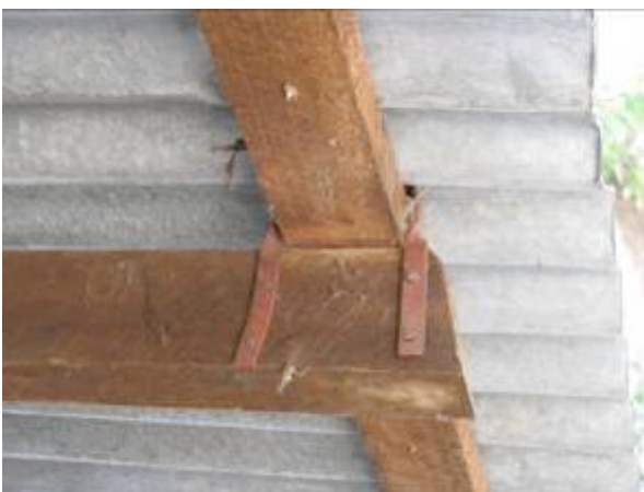
Purlin- rafter connection
