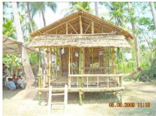
The Bamboo house model for the children to play and for the villagers to learn on construction technique
