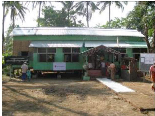
Atwin None Kaw School after strengthening
