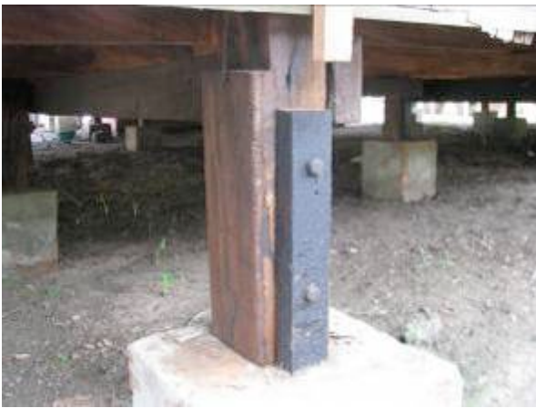
Post- Footing Connection
