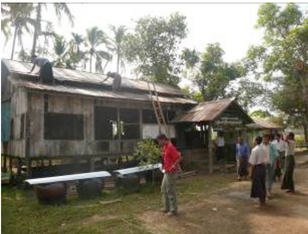
Atwin None Kaw School before strengthening
