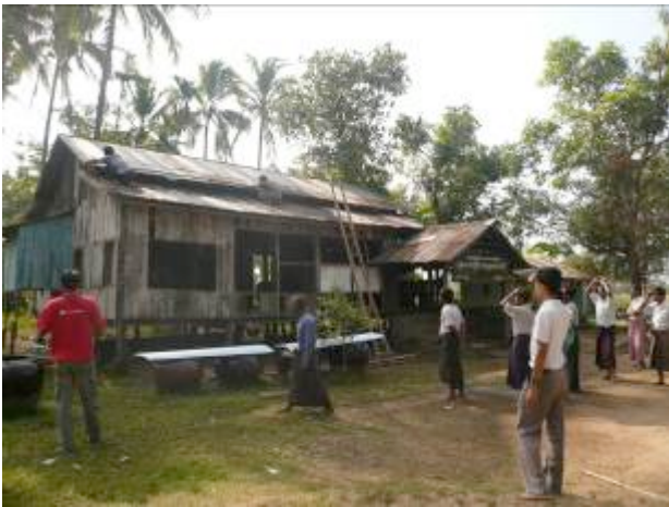
Atwin None Kaw School before strengthening
