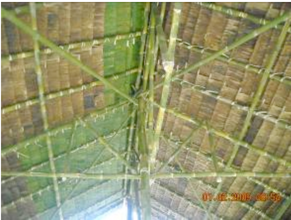
Bracing in trusses
