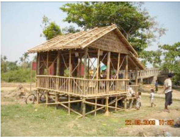
Bamboo House Model Framing
