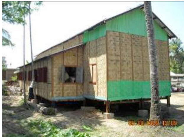
Atwin None Kaw School after strengthening
