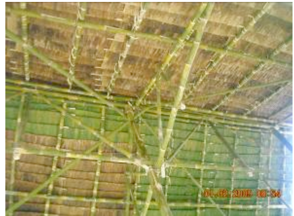
Diagonal bracing between trusses
