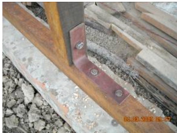
Cyclone strap in wall framing
