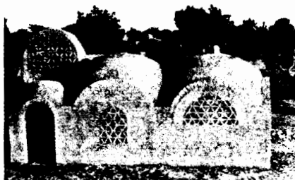
The recently constructed Literacy Centre was built in three weeks by locally trained builders. It covers an area 5m x 10m and uses mud-brick vault technology. The taller vault at the left, behind the entrance, is a wind-catcher. Photo: Allan Cain/Development Workshop.
