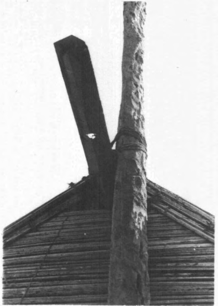
Detail of joint between central post and ridge pole showing gable end
