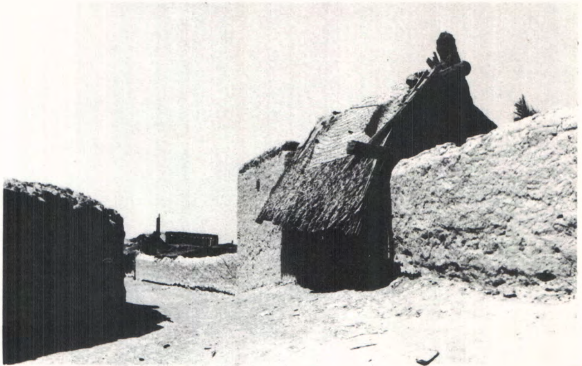
Fig 3.19 Winter Village Falaj al Qabael Note mud brick houses and added matting on barasti roof.
