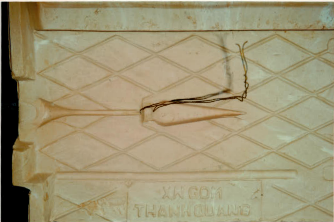
Fixing holes reintroduced into the underside of clay tiles, so that they can be tied down to battens with wires.
