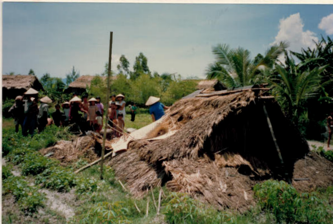
Damaged thatched houses after a small typhoon.
