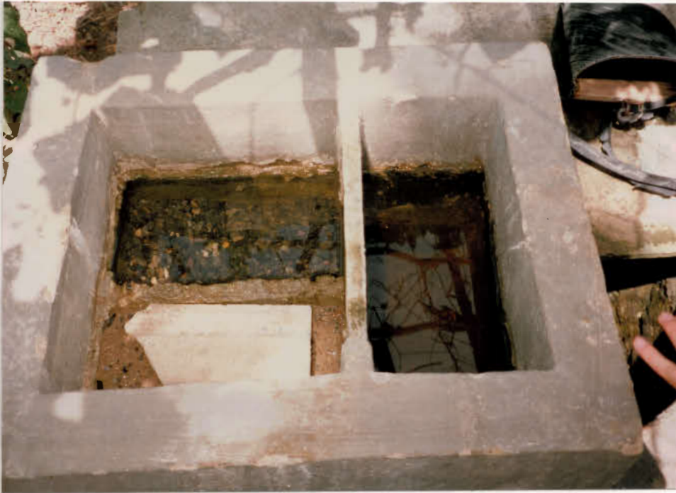
Water supply actions: family filters in Ninh Van
