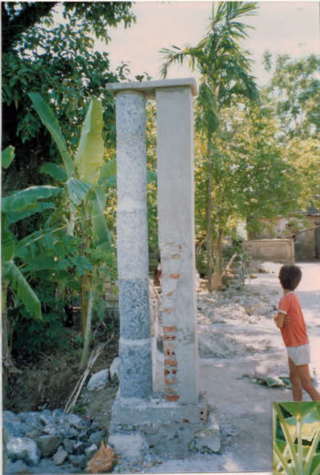
Building experiments - stone columns; semi dressed stone walls in Ninh Van
