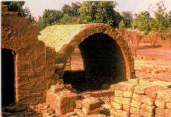
Above: a training-structure, on which the end-walls have been removed, shows the section of the Nubian vault. (Sevare, May '95)
