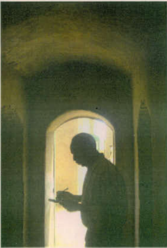
The construction of the toilets and showers used a narrow, shallow vault (see above) and small, flat, string-traced domes, so that with a minimum of infill, a flat roof could be achieved, (below) demonstrated by Ibrahim Tomota, the head mason for the site.
