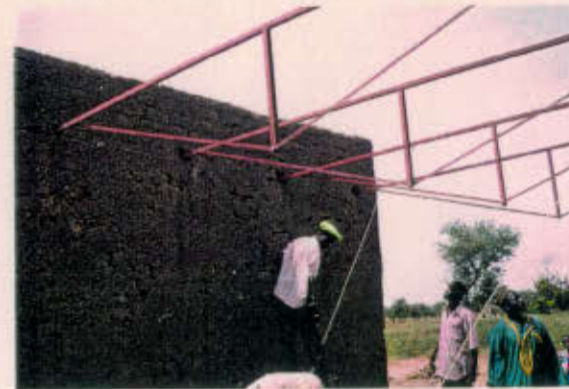
Right: 'hangar'-frame being erected at Soufourallaye- October '96
