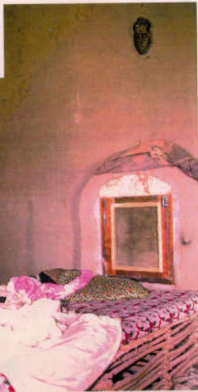
'Fireplace' inlet from windcatcher chimneys (at left) under construction and (below) when completed, with mosquito-screening.
