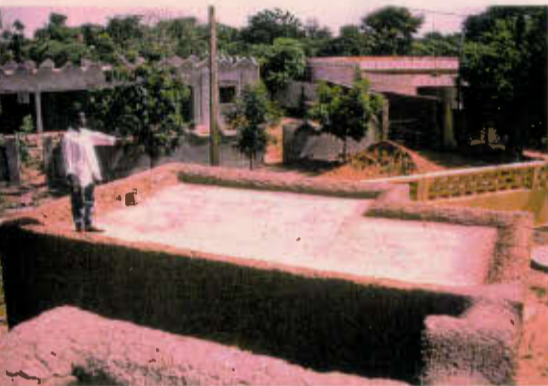
The construction of the toilets and showers used a narrow, shallow vault (see above) and small, flat, string-traced domes, so that with a minimum of infill, a flat roof could be achieved, (below) demonstrated by Ibrahim Tomota, the head mason for the site.
