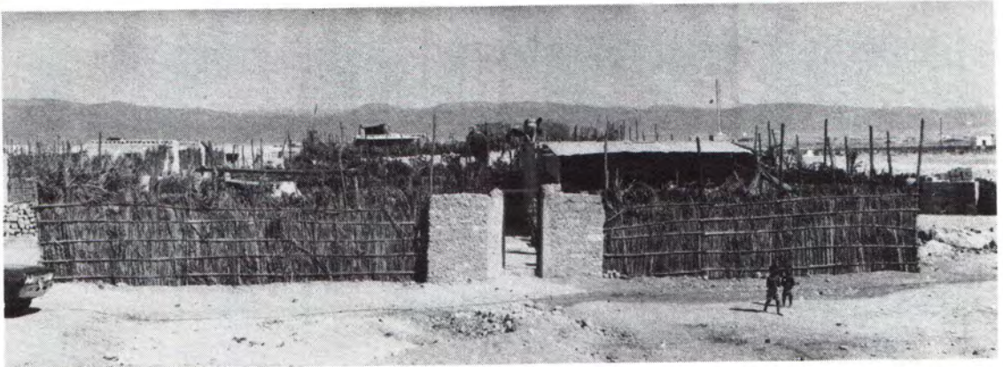
The first stage in owner built housing is the erection of a perimeter wall around the plot and the establishment of a formal entrance way.
