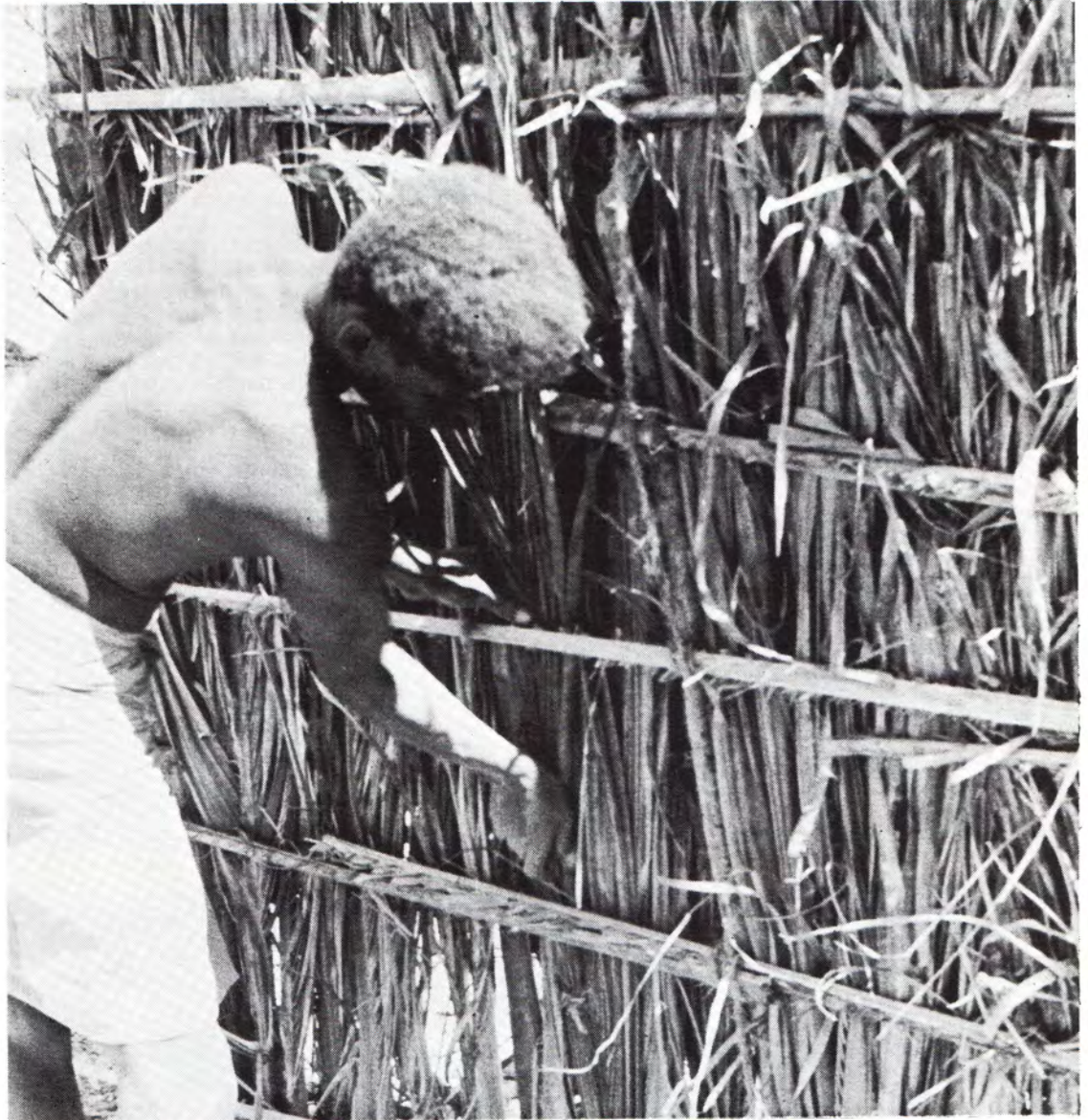
A framework of hardwood sticks or palm stems is the supporting structure for the walls. Leafy palm fronds become the screening material.
